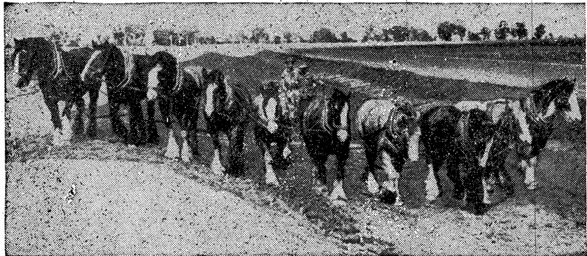
TEN HORSEPOWER IN ACTION . . . In these days of power-driven machinery, a ten-horse team is as rare as that day in June. This team is in use building an irrigation canal in the Murray valley soldier settlement, Victoria, Australia, where between 500 and 600 miles of irrigation channels are being excavated. The horses are used in preference to power machines because stamping of the horses' hoofs helps bind the soil on the banks of the channels. Notice the size and weight of the horses in this team. No wonder their feet bind the soil.
